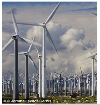
The windmills work in the same way as wind turbines, pictured. Blades are spun in the wind, which spins a shaft connected to a generator
